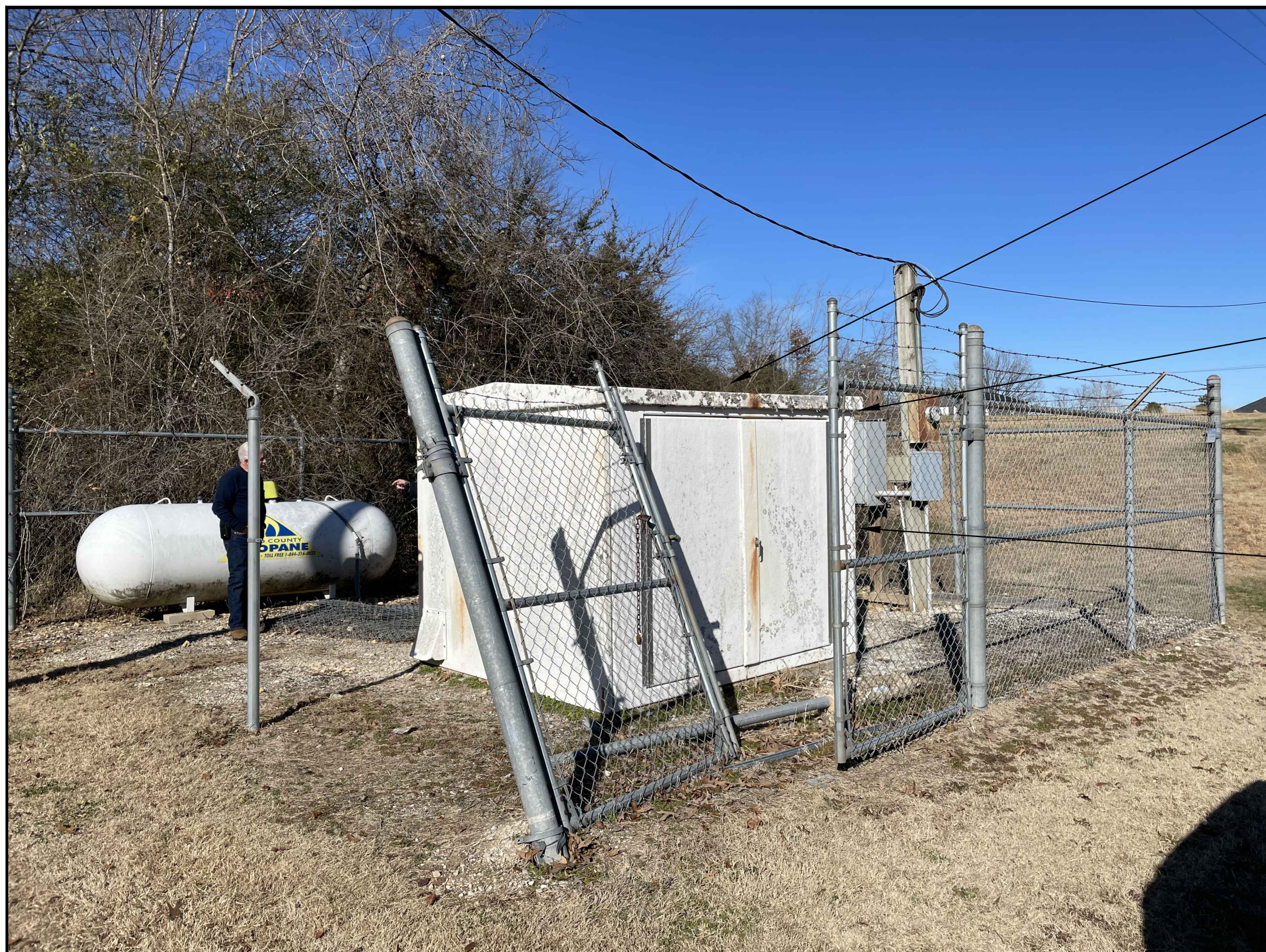
PHOTO HWY 9 S PS BUILDING NTS (A)
